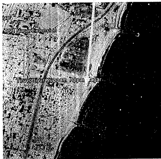
Fig.1 Aerial view of Thiruvottriyur Kuppam
